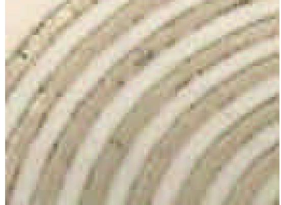
Figure 12: Cracking of the Paste Due to the Method Employed.
