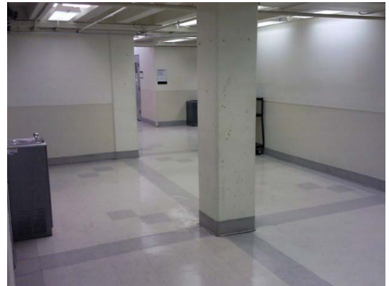
Figure 13: Mapped Area in Towne Building Hallway (Part 2, back-right)
